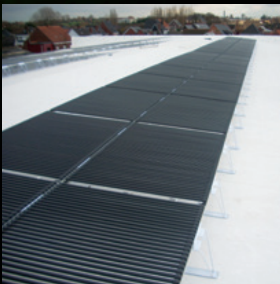
Industrial building (Belgium)
