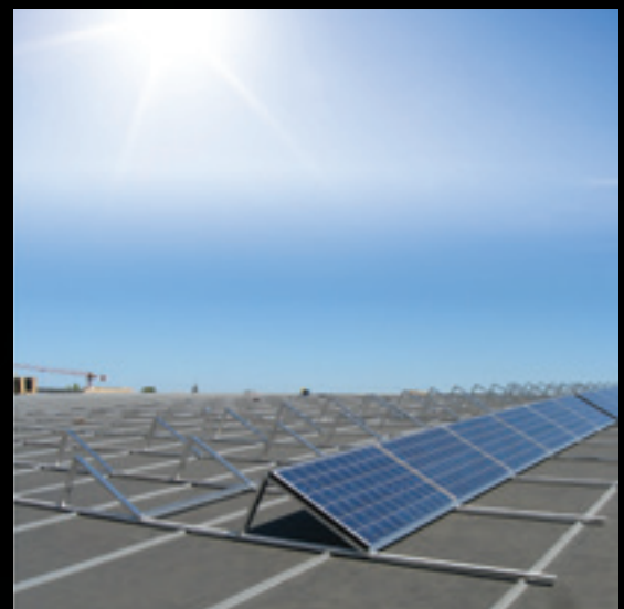
Industrial building (Belgium)
